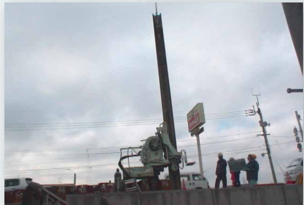
Steel sheet pile pull-out situation
