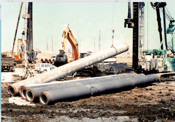
Negative friction force countermeasure pile construction status.
