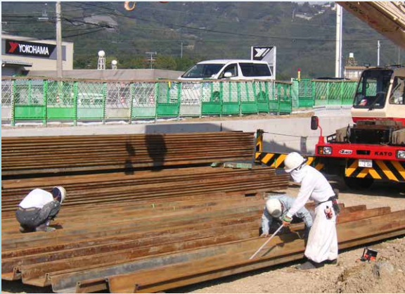
Laying and cleaning
