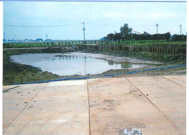
Photograph-14 Sand guards method of construction.
