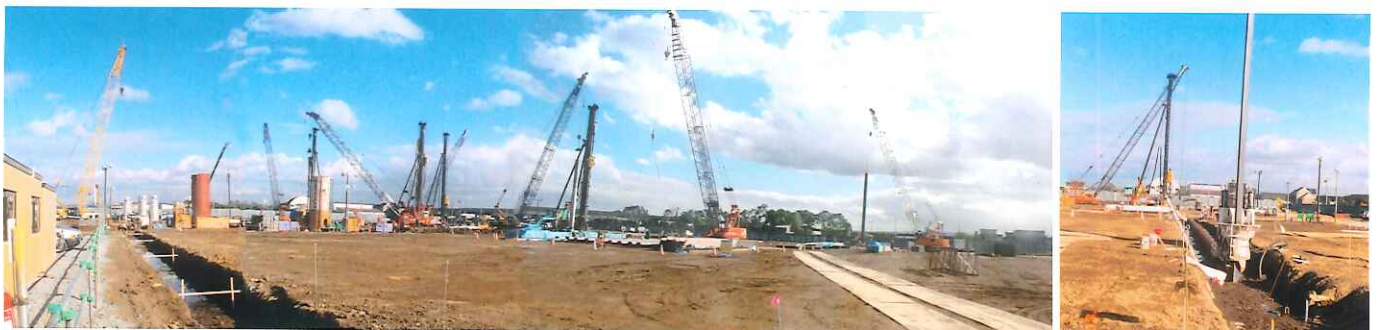
Photograph-16 A water sealed wall method of construction.
