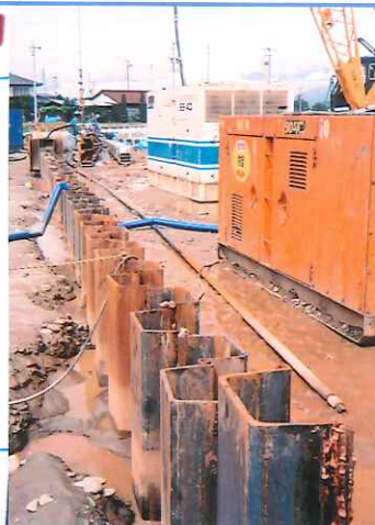
Photograph-15 A water sealed wall method of construction.
