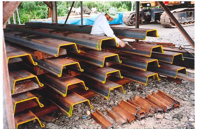
Photograph-4. The example of the way of putting steel sheet-pile.
