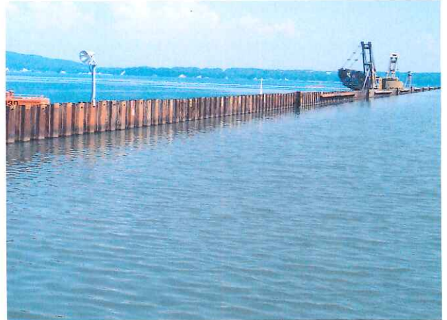
Photograph-11 A deadline method of construction.
