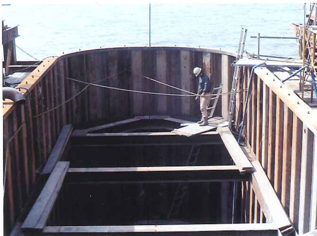
Photograph-12 A caisson foundation.
