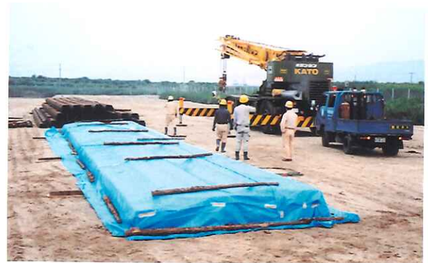
Photograph-6. Cure (drying)
