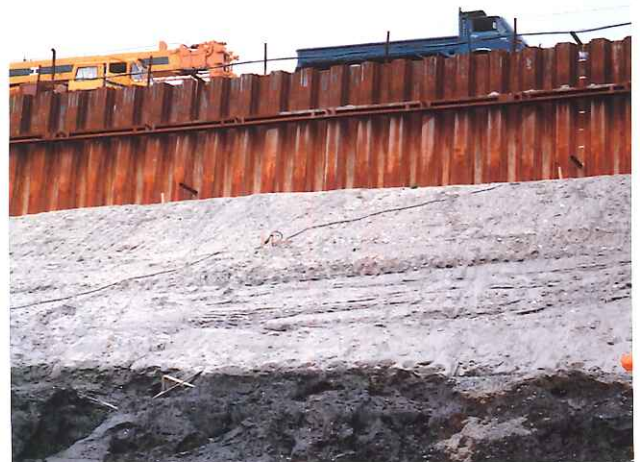
Photograph-13 Sand guards method of construction.
