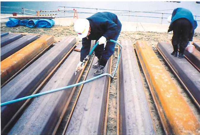
Photograph-3. Air blow.
